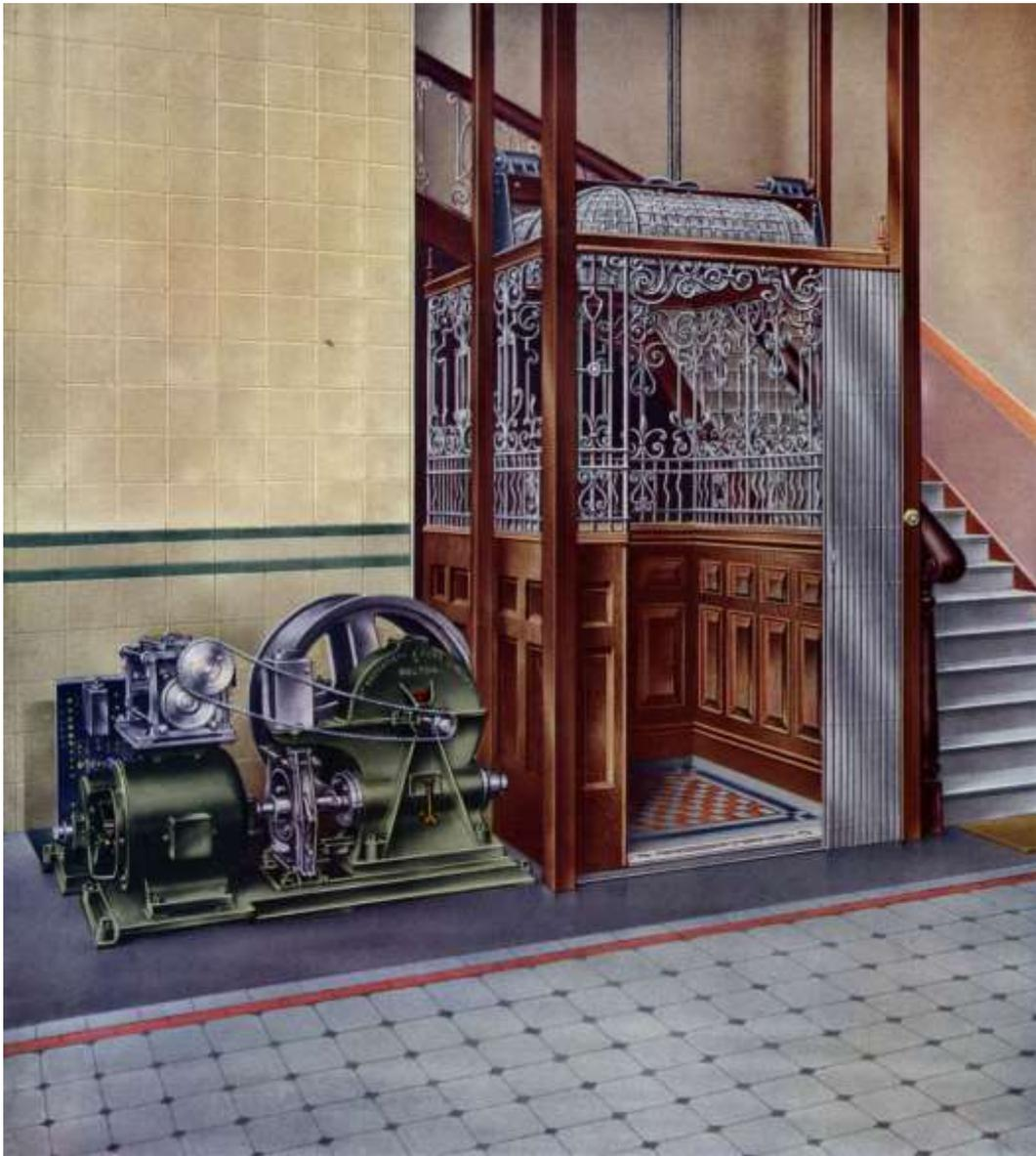
**Figure 15 Lift Engine & Car, *Wadsworth's Lifts, Transporters, Hoisters* (c. 1930)**
