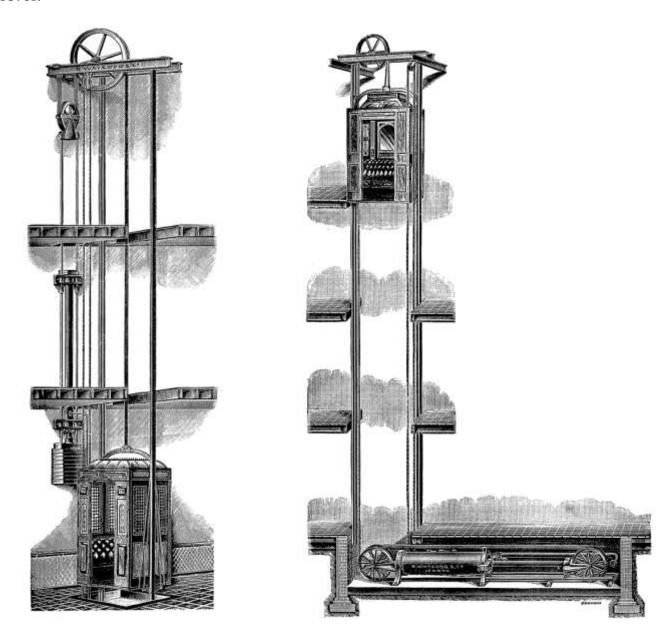
Figure 4 Waygood's High Pressure Suspended Lift (right) & Low Pressure Suspended Lift (left)
