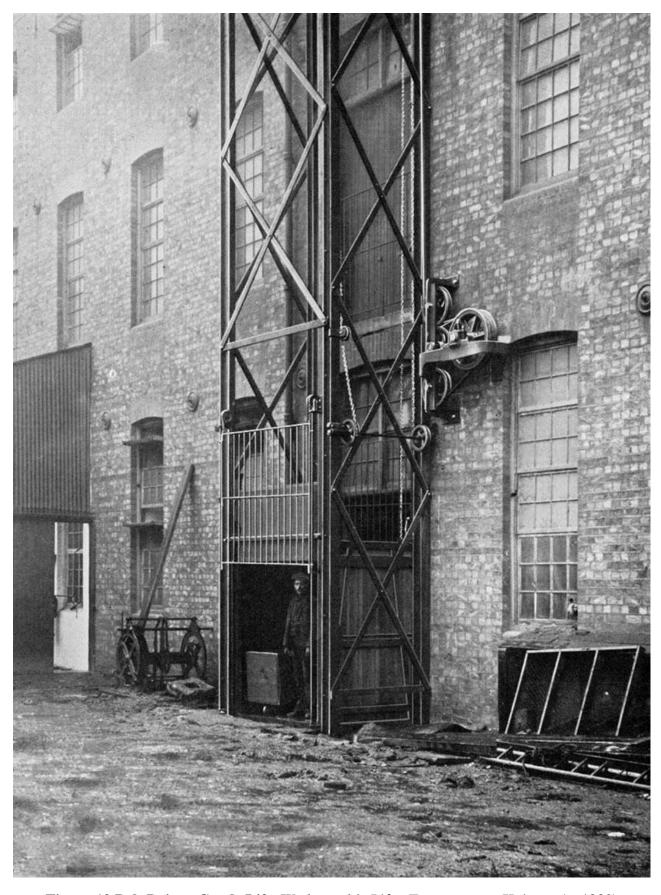
Figure 19 Belt Driven Goods Lift, Wadsworth's Lifts, Transporters, Hoisters (c. 1930)
