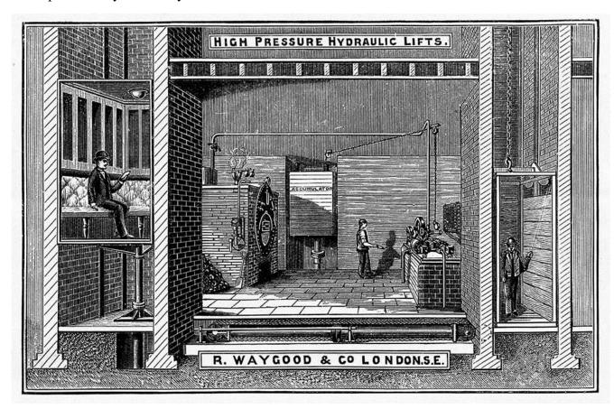
Figure 5 Waygood High-pressure Hydraulic Plant
